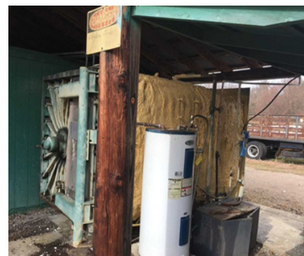
North Carolina's decontamination unit.
